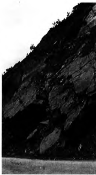
Photo- 4. A planar failure at 77 km stone along the road
